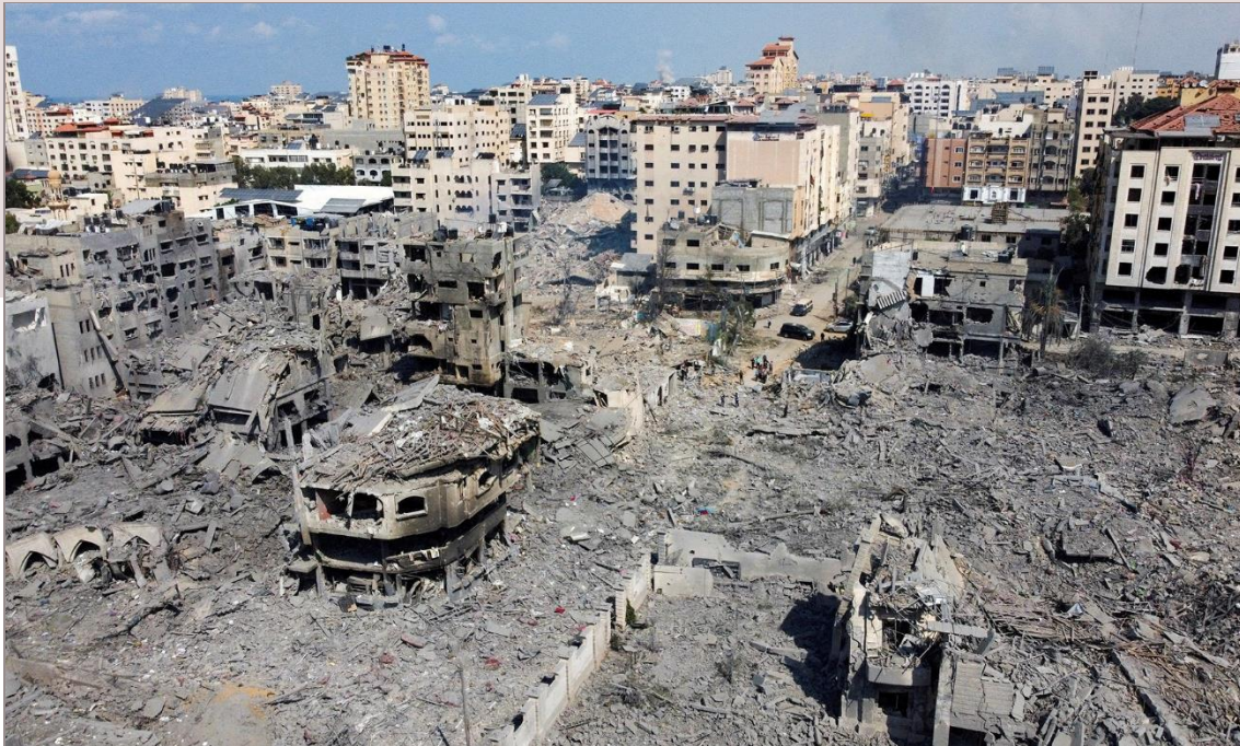
The magnitude of damage in Gaza (Al Jazeera)
